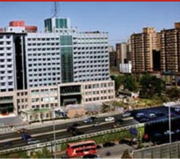
Beijing Traffic Control Center Headquarters
