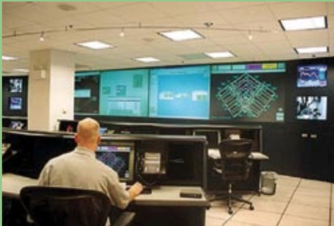
The Pentagon Building Operations Command Center
