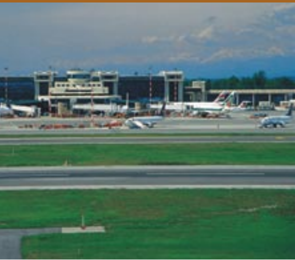
Malpensa Airport in Milan, Italy
