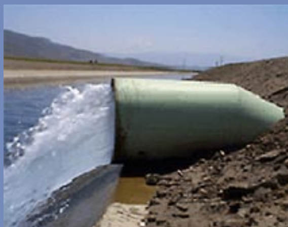
Water Transfer from Ground Storage
