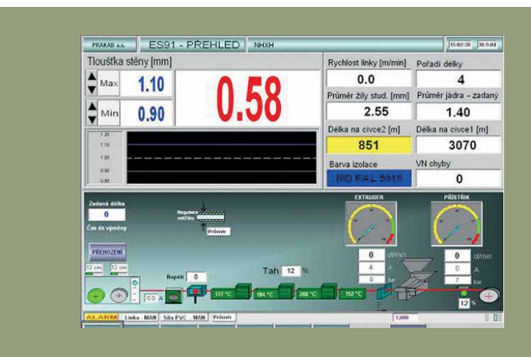
Main Control Screen at PRAKAB a.s.
