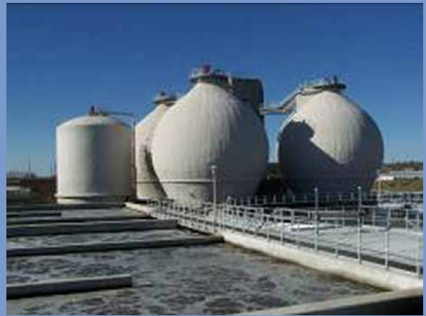
Anaerobic Digesters
