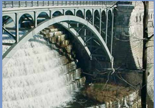
Water from the New Croton Reservoir Travels 24 Miles Before Entering NYC Via the Bronx
