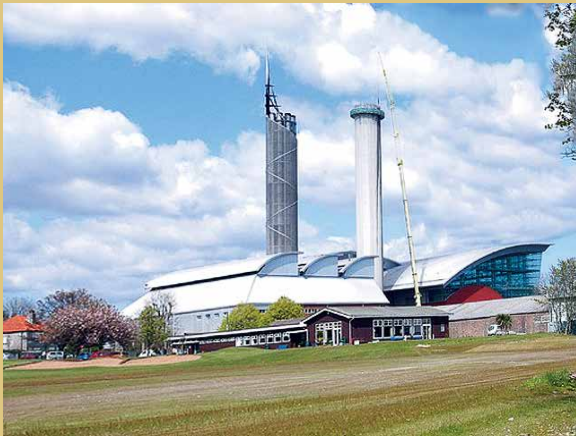
Pulrose Power Station
