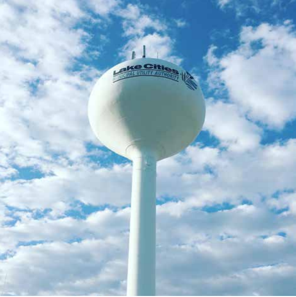
Webb County Water Treatment Plant Rio Bravo, Texas
