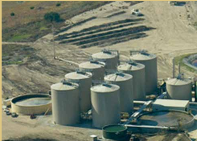
Microgy's Huckabay Ridge Facility in Texas
