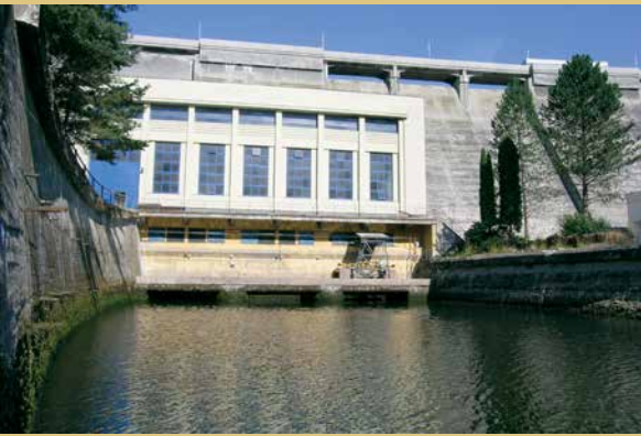
An E.ON Hydroelectric Power Plant
