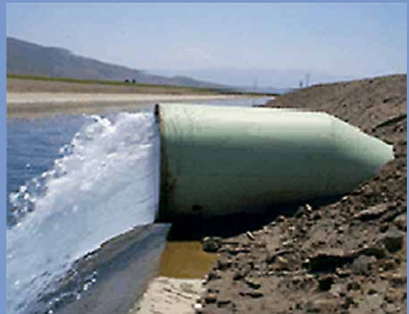
Water Transfer from Ground Storage
