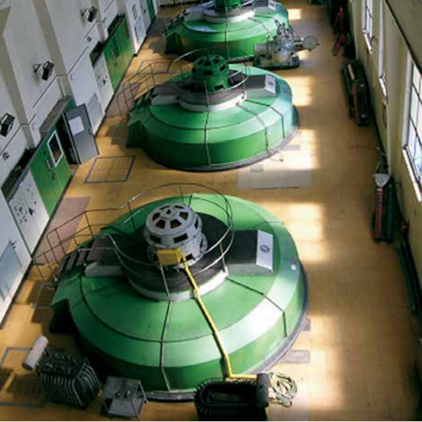
Hydro Turbines E.ON Hydro Power Station
