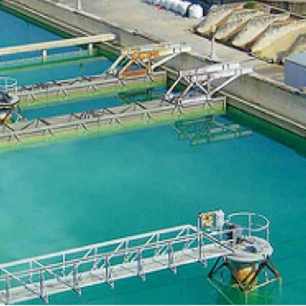
A Water Processing Facility at Hyderabad Water Supply & Sewerage Board
