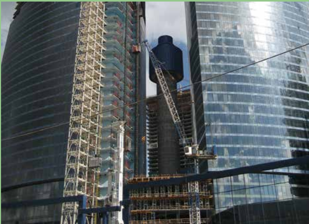
The Federation Tower Under Construction Moscow, Russia
