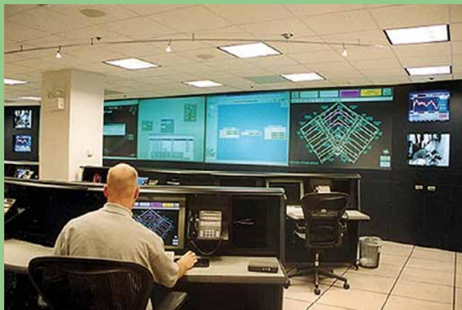
The Pentagon Building Operations Command Center
