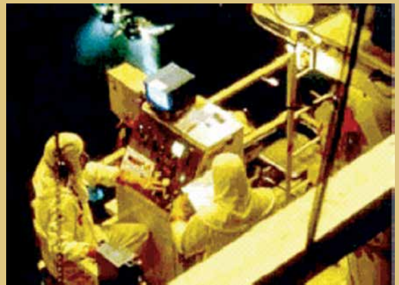
Operators at Refueling Machine Controls
