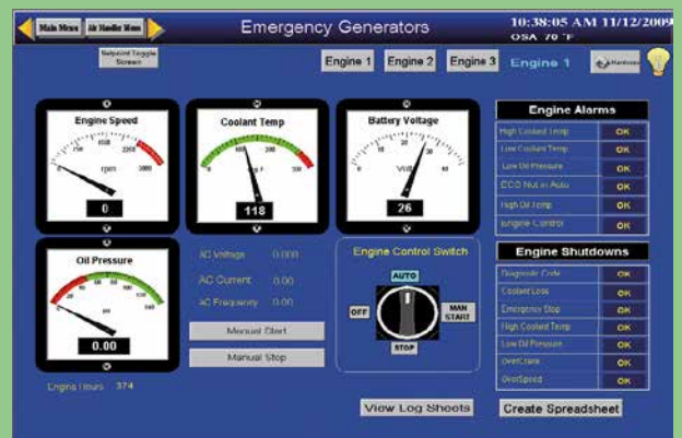
View of Emergency Generators
