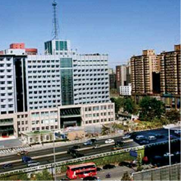
Beijing Traffic Control Center Headquarters
