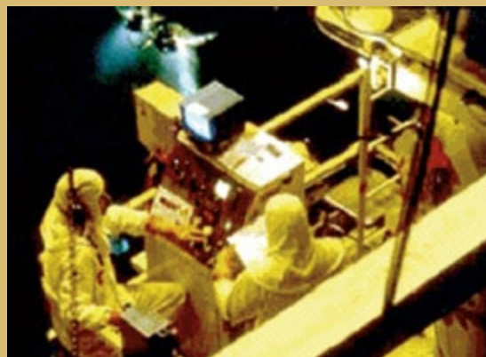
Operators at Refueling Machine Controls
