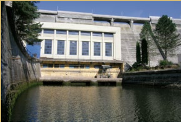
An E.ON Hydroelectric Power Plant
