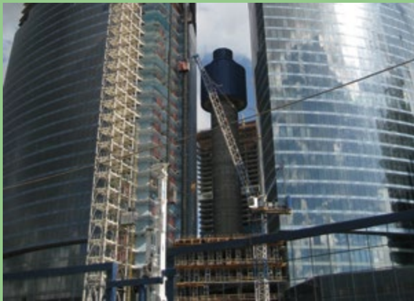
The Federation Tower Under Construction in Moscow, Russia
