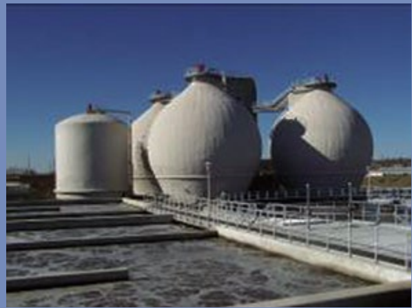
Anaerobic Digesters
