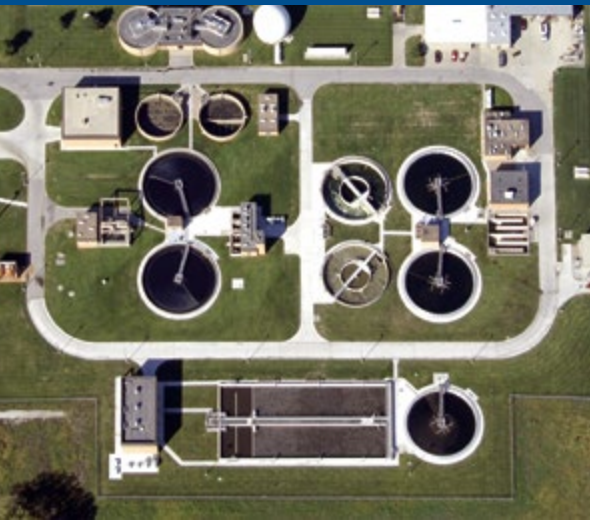
Lincoln Wastewater System's Northeast Treatment Plant
